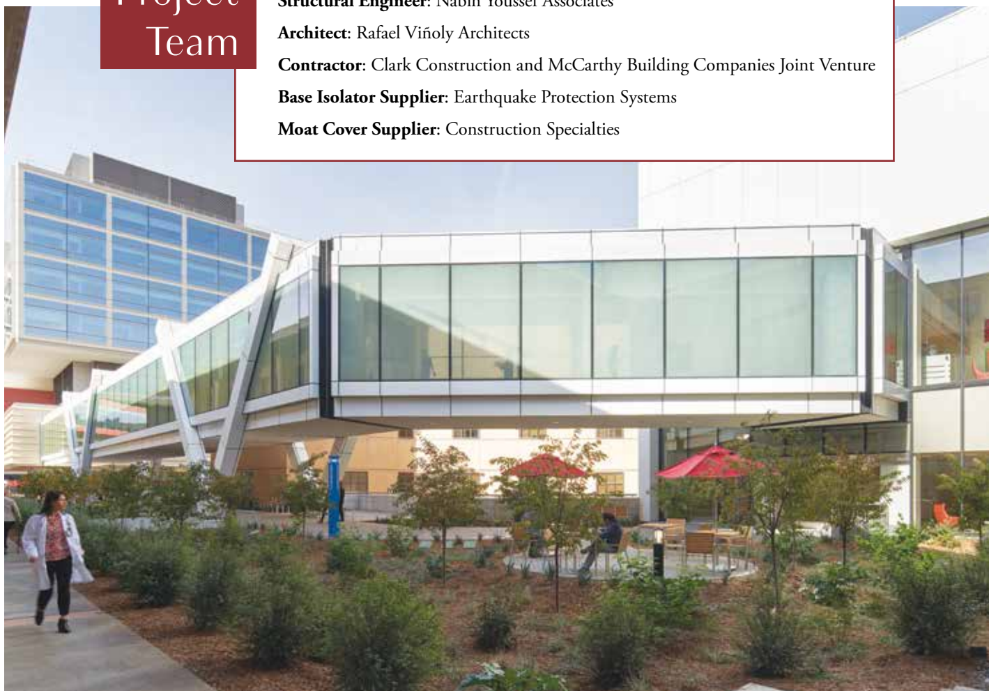
Figure 4. Skybridge connecting the new base-isolated hospital to an existing building. Courtesy of Bruce Damonte.
