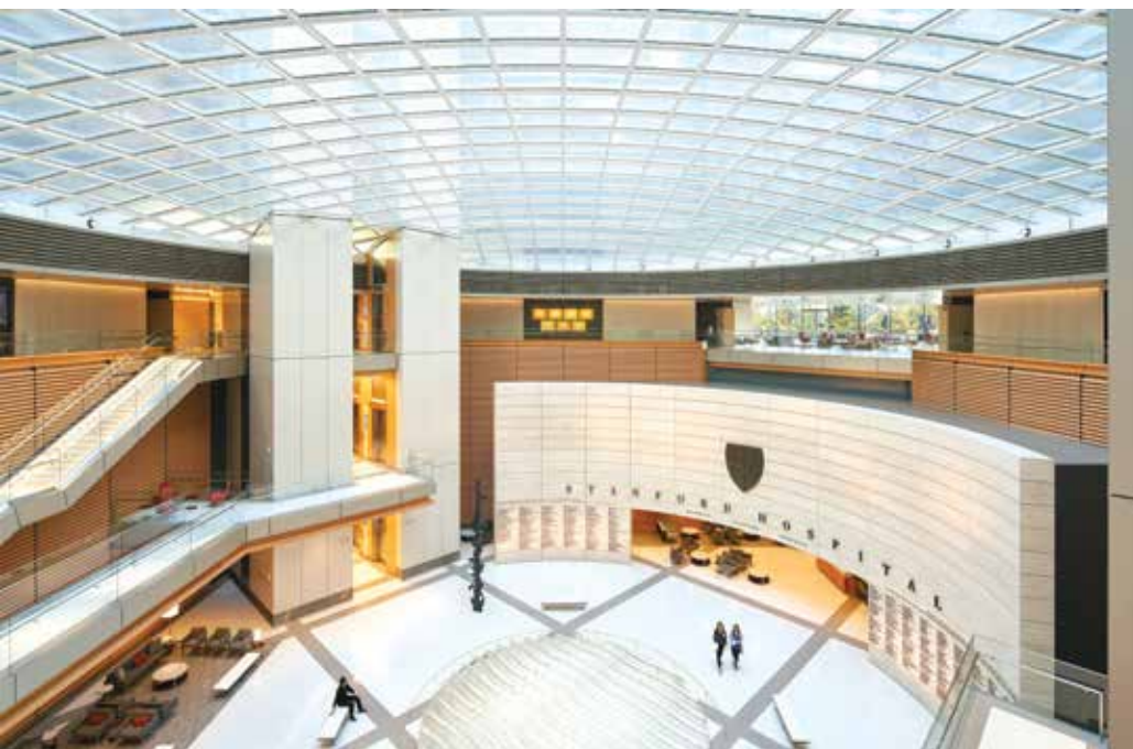
Figure 2. A view of the gravity-defying 120-foot-span dome skylight over the central atrium. Courtesy of Bruce Damonte.
