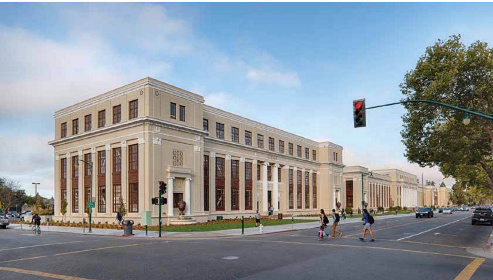
Looking down Central Avenue.
