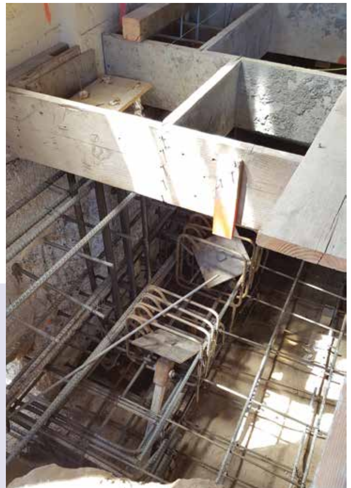
Top of battered helical piles at pile cap.
