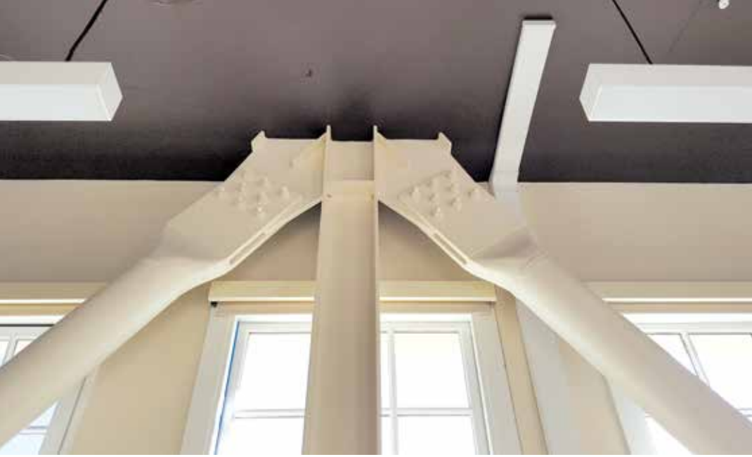
Cast Connex HSC brace connection.
