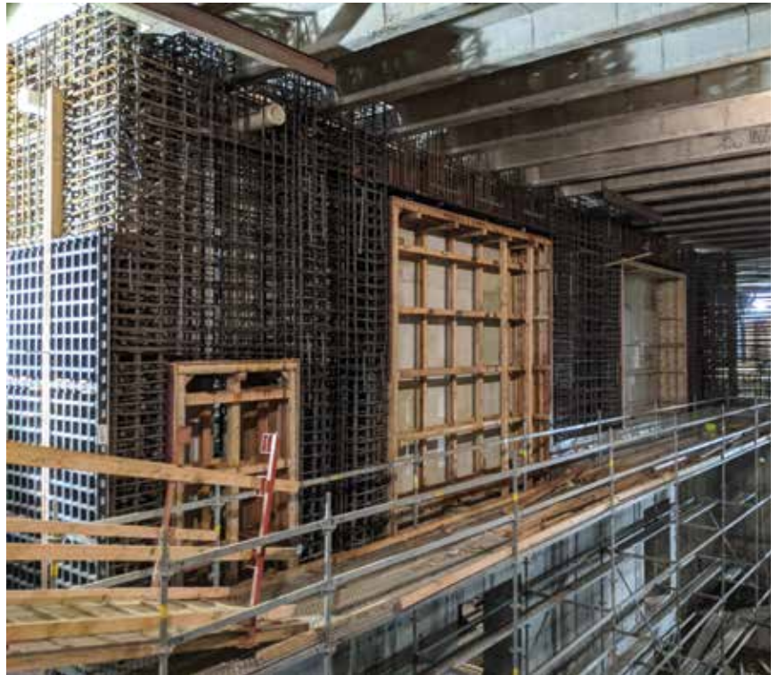
Figure 5. North-South core wall reinforcing.
