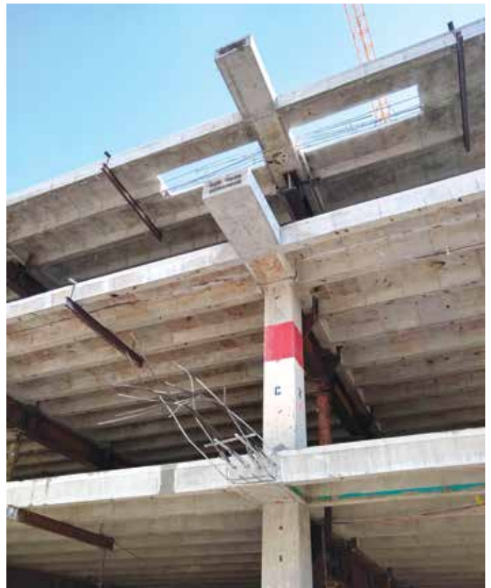
Figure 4. New cantilevered girder ends at various stages of construction, with continuous shoring installed.
