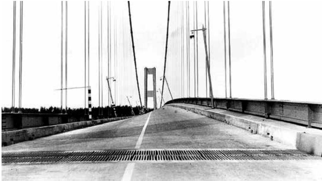
Tacoma Narrows Bridge twisting prior to collapse.
