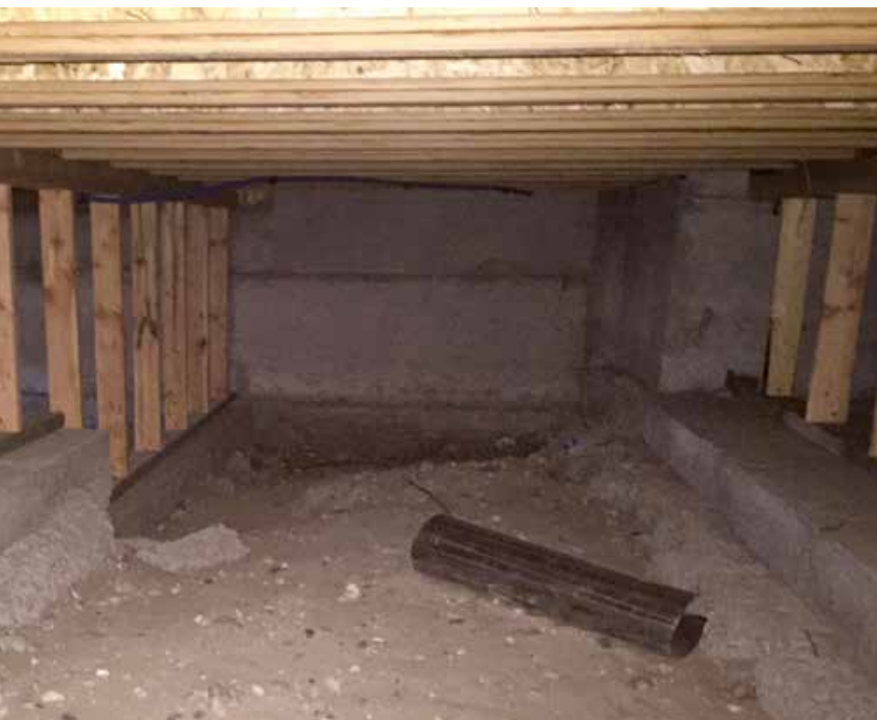
Figure 5. Interior cripple walls.
