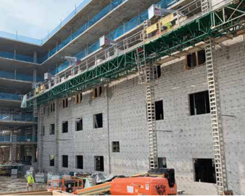
Figure 4. Masonry construction using MULE.
