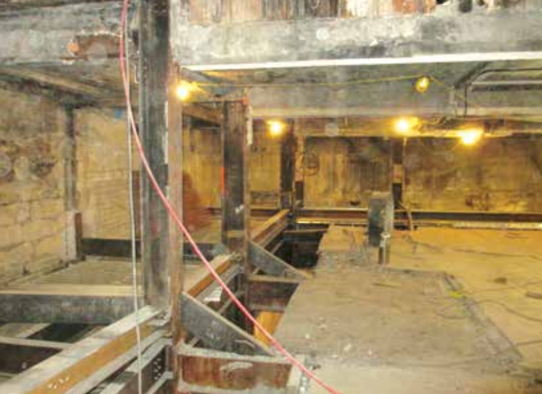
Figure 3. Cellar column temporary bracing.
