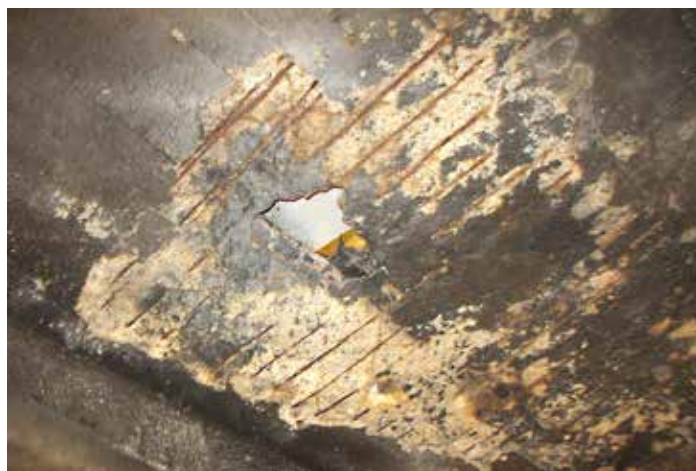
Figure 2b. Cellar slab deterioration
