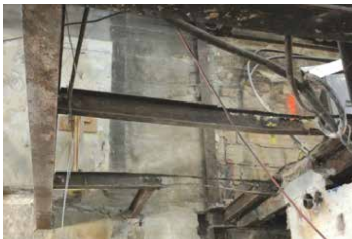
Figure 2a. Section loss at corroded cellar steel beams
