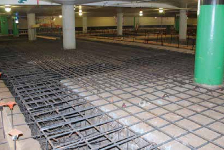
Figure 5. Foundation strengthening in the form of combining multiple existing spread footings.
