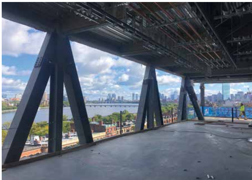
Figure 6. Truss framing at floor level.
