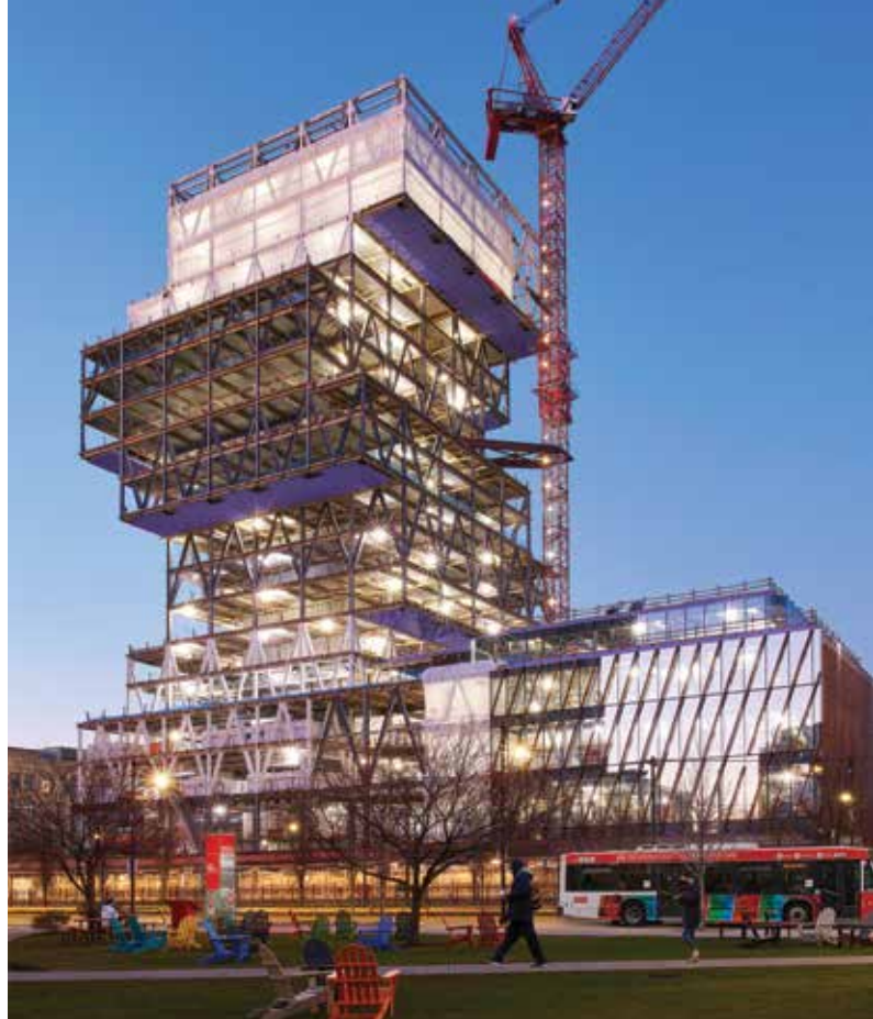
Figure 7. Steel framing. Courtesy of John Cannon.
