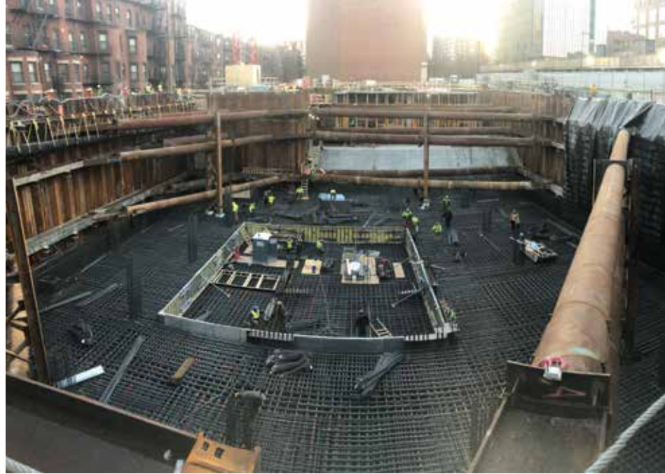
Figure 3. Tower mat slab construction.
