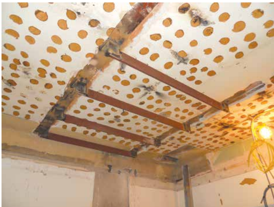
Figure 20. New steel angles installed first at the arch span adjacent to the new chute and chase openings.
