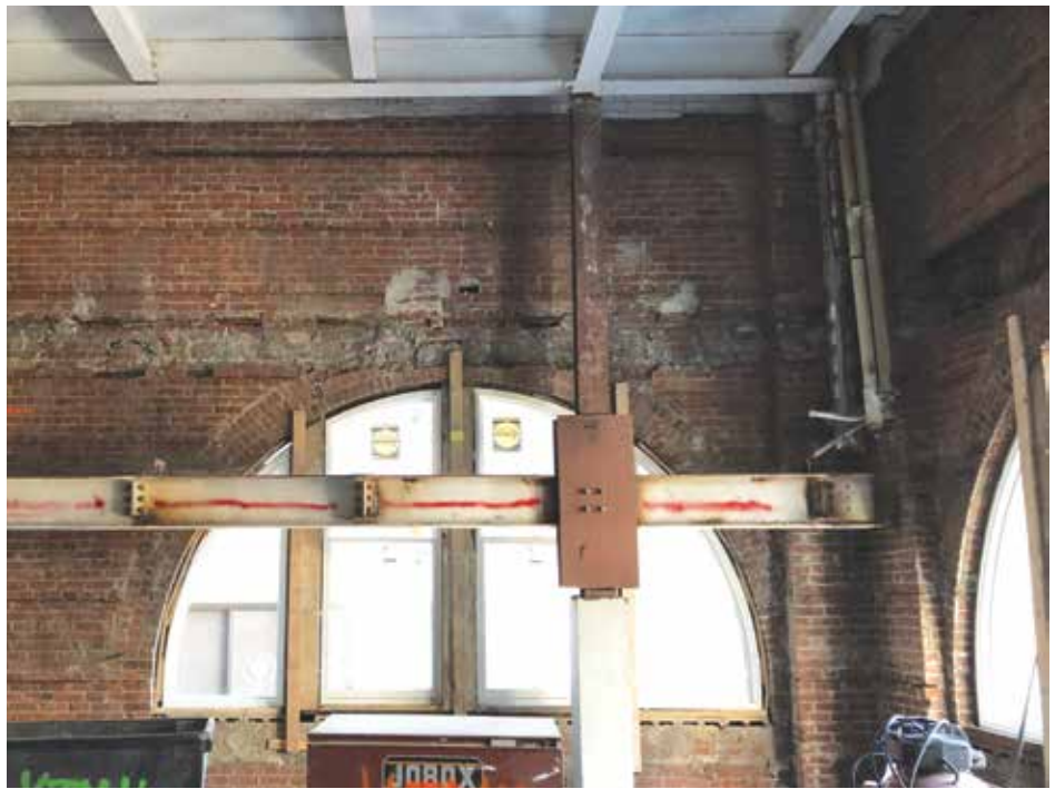
Figure 21. Reinforced discontinuous column at 2 nd -floor mezzanine cantilevered beam.
