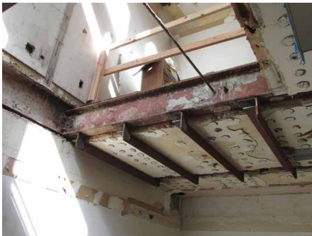
Figure Q. Existing arch tie rods at the new chase and chute openings.
