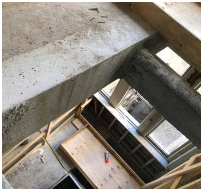
Figure 19. New cast-in-place concrete beam at new openings in the arch floor to replace damaged tile.
