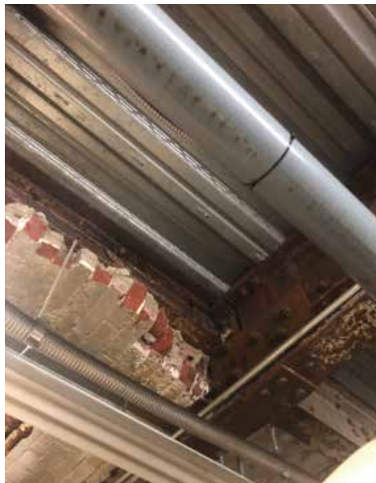
Figure 22. Existing 20-inch-deep, Carnegie Steel B3 transfer girder splice.
