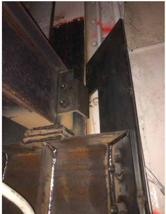
Figure 18. 1 st -floor loft beam connection to existing Gray column.
