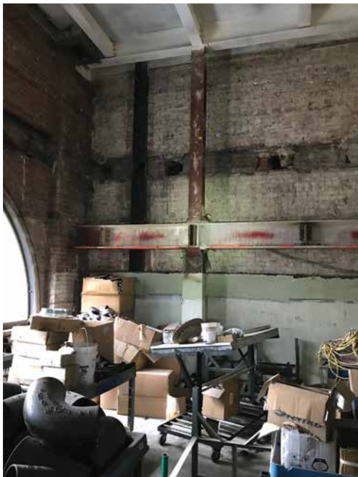
Figure R. Remaining 2 nd -floor mezzanine cantilevered beam and discontinuous column.
