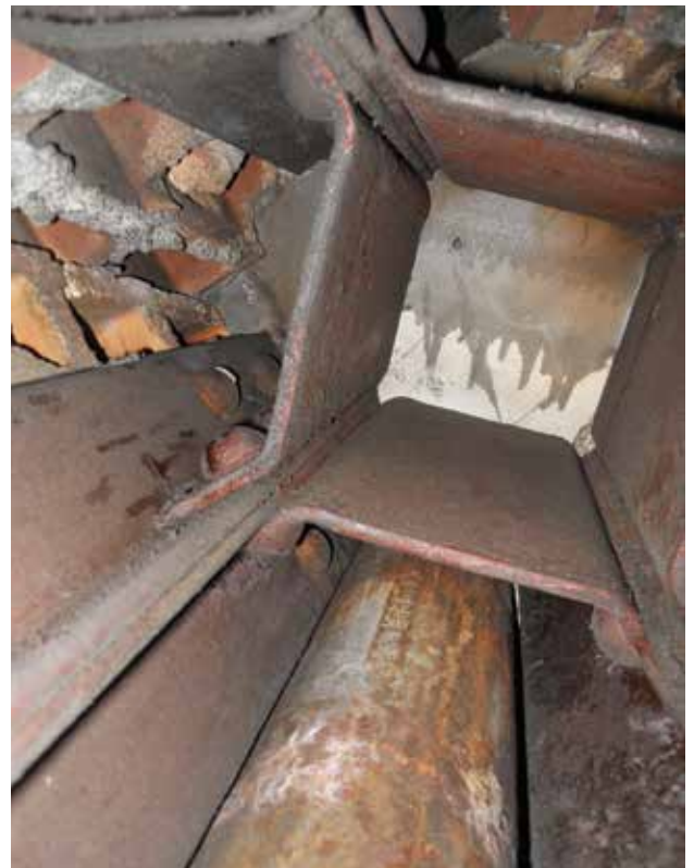
Figure 16. Riveted gusset plate connectors at the Gray column vertical double angles.
