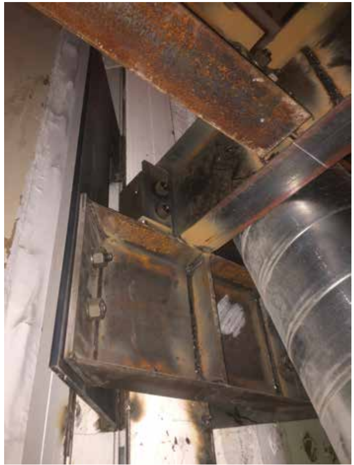
Figure 17. 1 st -floor loft beam connection to existing Gray column.
