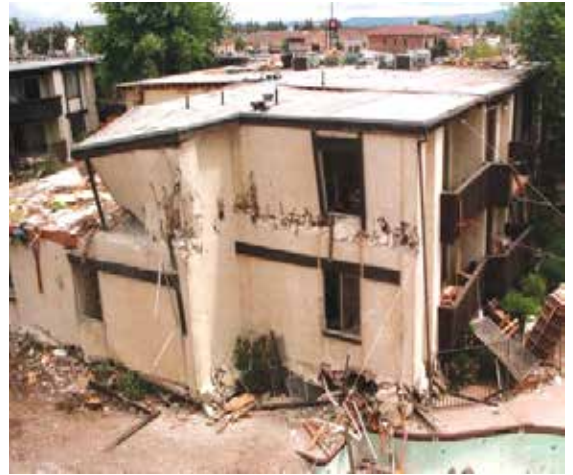
Northridge Meadows Apartments after the 1994 Earthquake.
