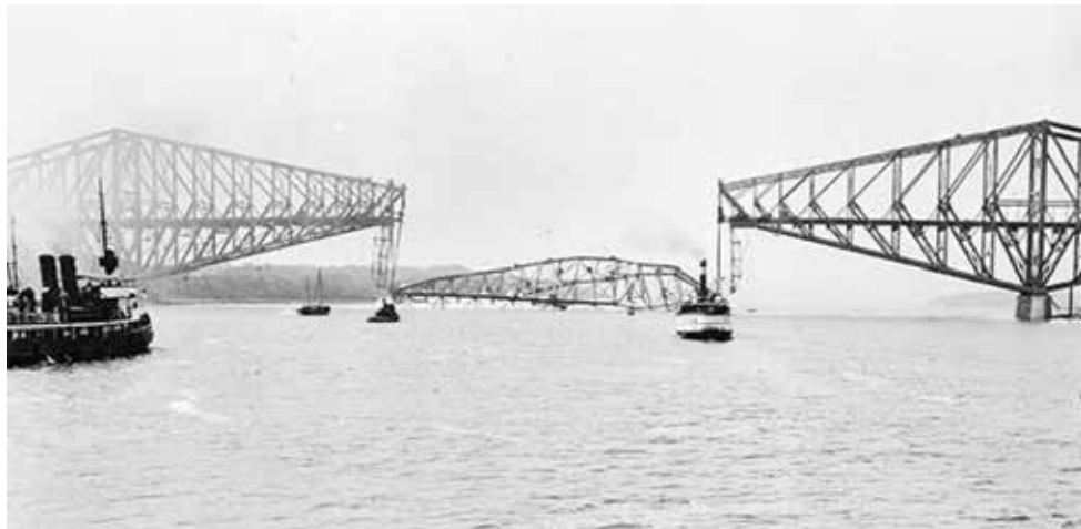
Suspended span collapsing into the St. Lawrence River.
