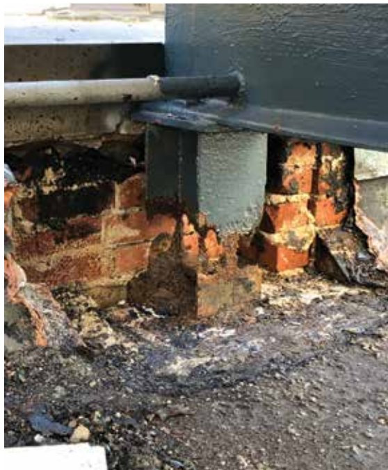
Figure 14. Corrosion and excessive section loss at an existing cooling tower steel dunnage column support.
