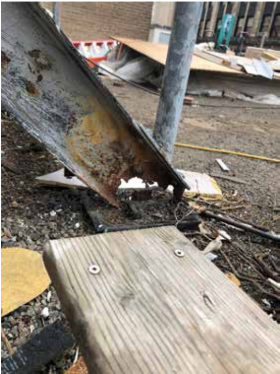
Figure N. Corrosion and excessive section loss at the additional mechanical penthouse exterior stair stringer.
