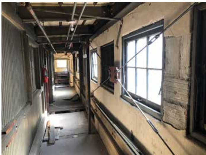
Figure 11. New vertical X-bracing at mechanical penthouse.
