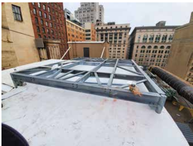
Figure K. Mechanical penthouse high roof RTU support steel dunnage frame.
