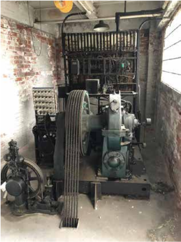
Figure O. Existing Otis freight elevator machinery.
