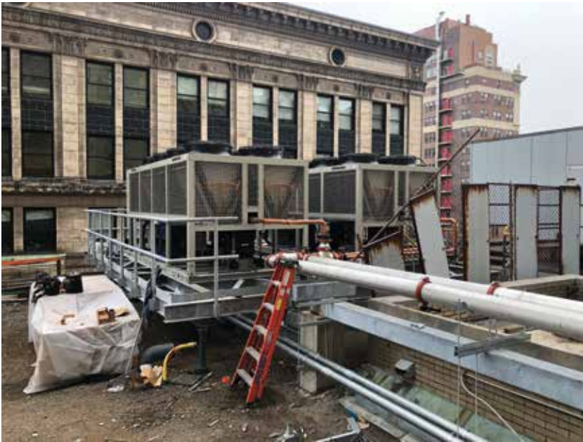
Figure M. Completed chiller dunnage framing (not including grating) and pipe support frame.
