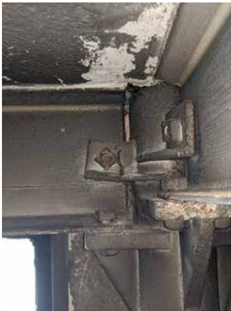
Figure 13. Cracked beam-web connection clip at a penthouse cast-iron column.
