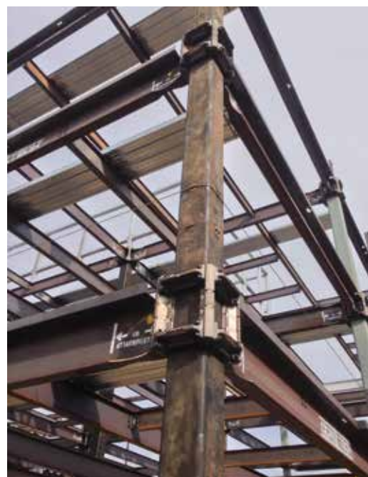
Figure 5. Framing at ConXtech corner column.
