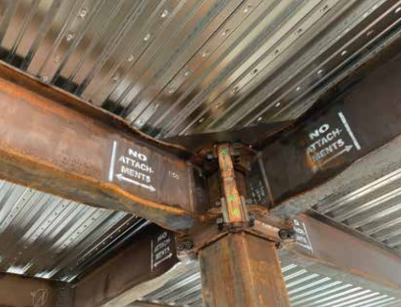
Figure 3. ConXtech bi-axial bolted moment frame connection.
