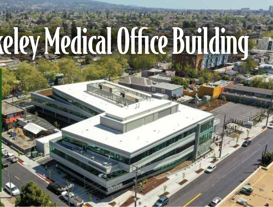
Figure 1. Aerial view of the building (looking southeast).
