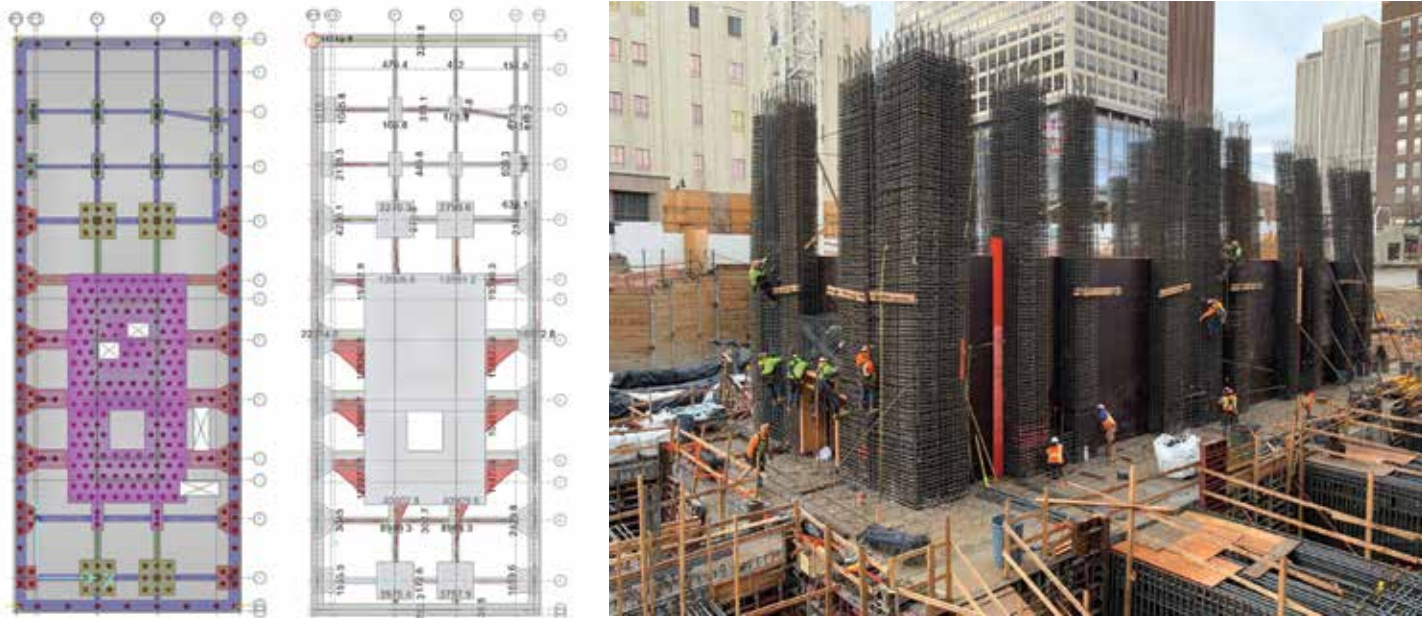
Figure 4. Plan of foundation model, outrigger grade beam moment diagram, and core wall mat foundation.
