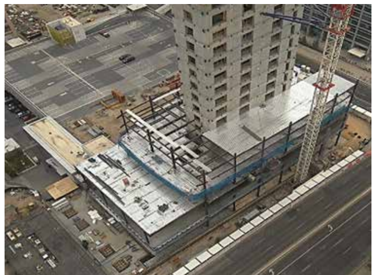
Figure 7. Construction of core walls and steel at Level 6.
