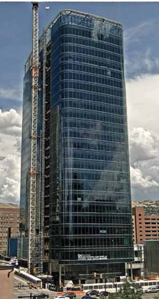
Figure 1. 95 State nearing completion in late 2021.
