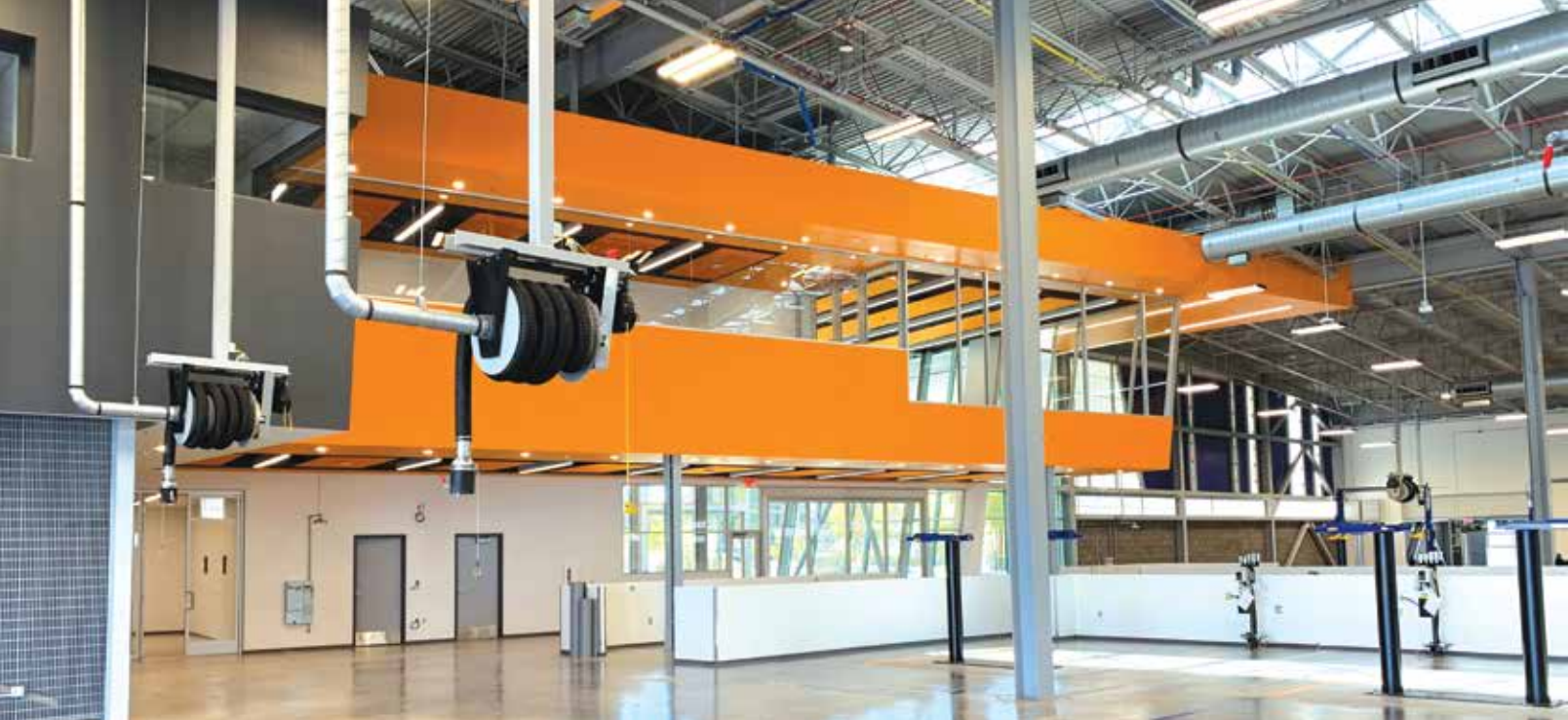
Hose reels cantilever from the 50-foot high roof.
