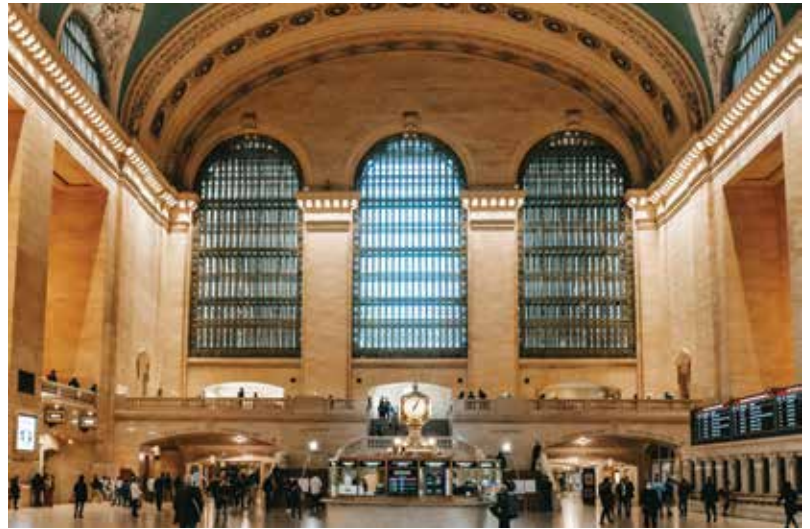
Archaic building materials may present challenges in determining the fire resistance of structural elements.
