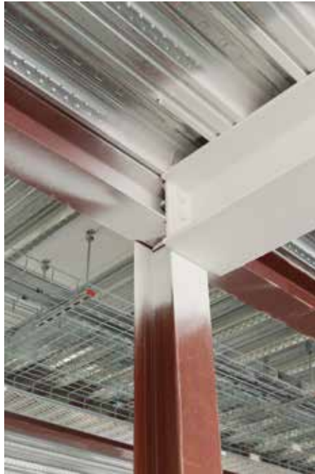
Intumescent coatings can be used to achieve required fire resistance for structural members.
