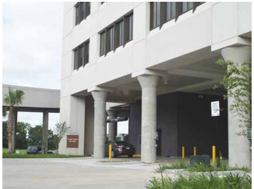
Figure 5. The Plaquemines Parish new medical center patient care areas are 23 feet above grade. Emergency vehicle ramp (background) provides direct access at the second level.
