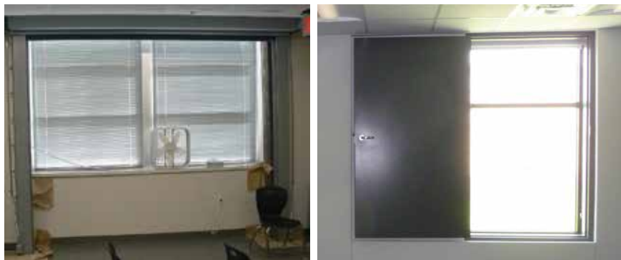
Figure 4. Different configurations of protective shutters (rolling and swinging).
