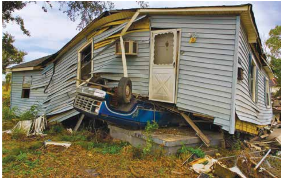
Figure 1. Extreme storm damage.
