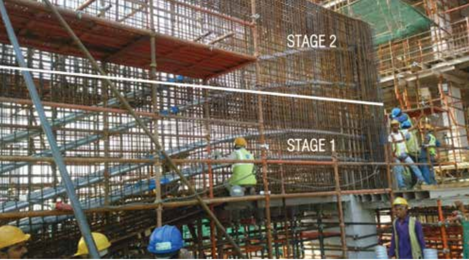
Aperture transfer girder.
