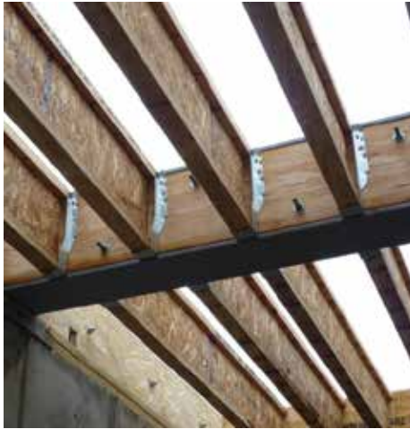
Prefabricated wood I-joists.
