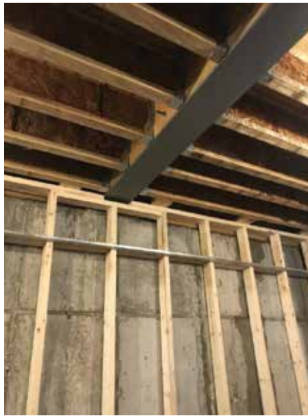
Wood joist connection at steel beam.
