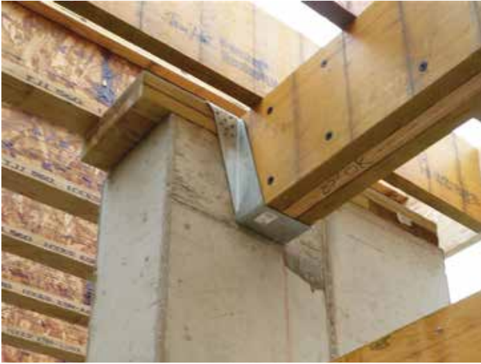
Custom wood connection at a concrete wall.
