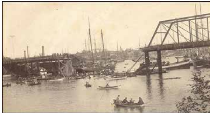
Failed 150-foot span, search for bodies underway.
