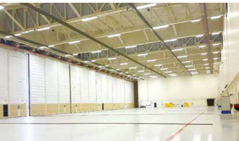
Figure 1. Interior of the completed hangar bay.
