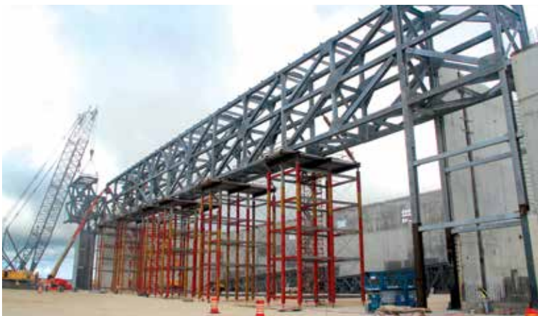
Figure 4. Box truss during construction.
