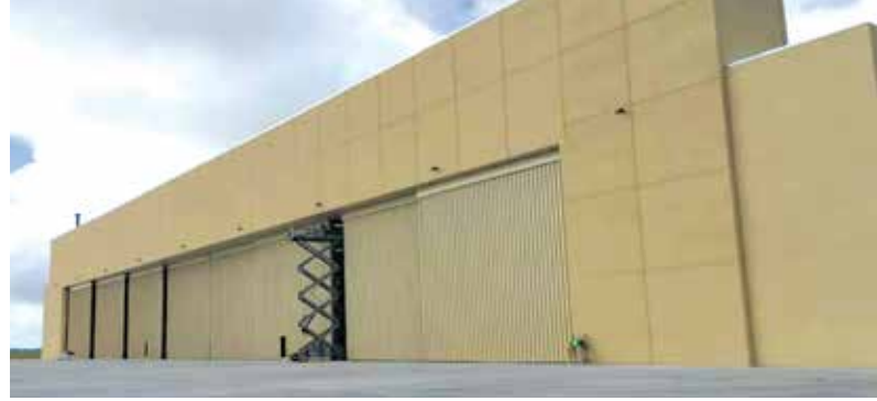
Figure 3. South elevation of the completed hangar.
