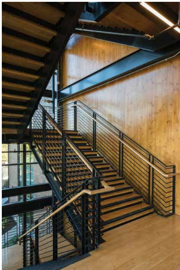
Figure 2. CLT stair shaft. Courtesy of Lara Swimmer Photography.
