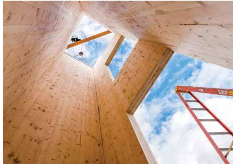
Figure 1. CLT elevator shaft.
