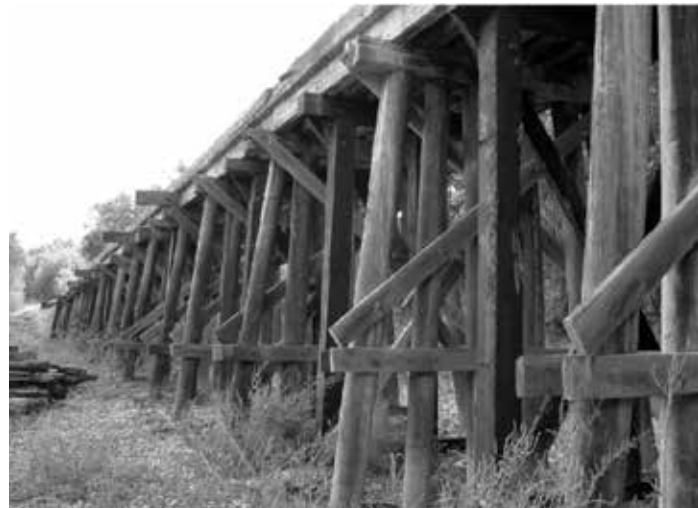
Inverted W wooden trestle with piles, similar to Blackshear.
