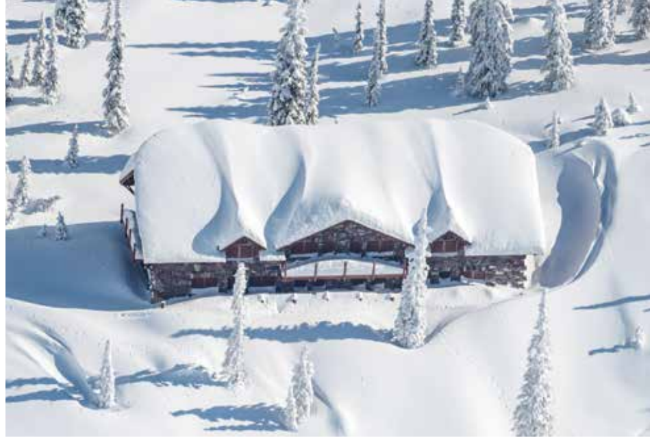
Figure 10. The roof endures its first load test after the first construction season. Courtesy of Gravityshots.com.
