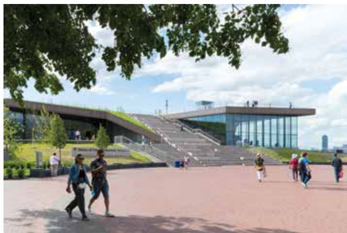
Helping to build a museum on tiny Liberty Island is no ordinary task. High Concrete Group manufactured and erected 83 pieces of precast concrete for the striking building. Credit: Iwan Baan, courtesy of FXCollaborative.
