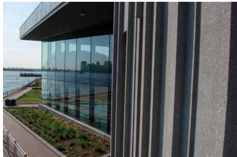
High Concrete Group shared Tekla models showing how the panels would connect to the steel frame.
