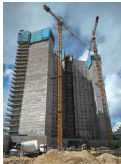
Tower nearing completion of the structure.
