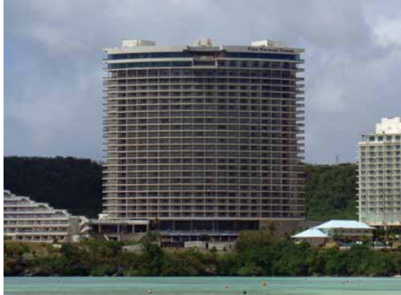
Topping off of structural framing.
