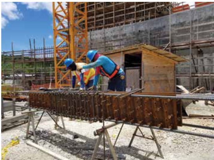
Composite coupling beams being prepared for installation.
