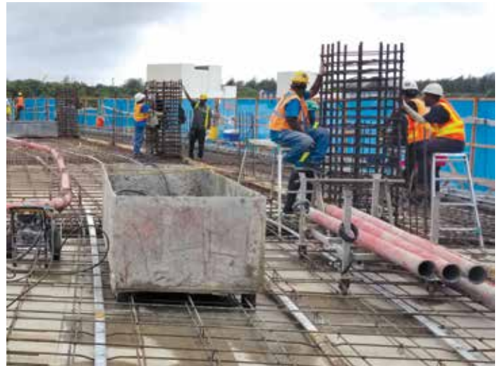
Bonded post-tensioning placed along the arc of the floor slab.
