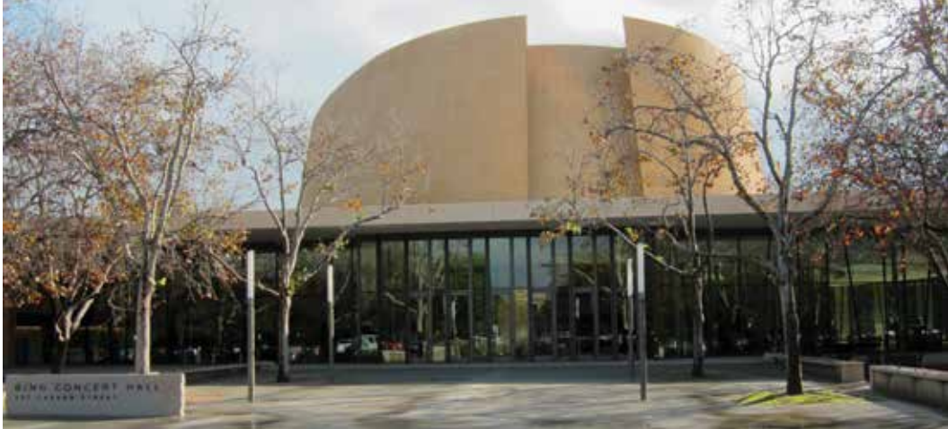
Bing Concert Hall – Stanford University. A shotcreted truncated cone. Courtesy of Joseph J. Albanese, Inc.
