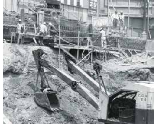
Shooting a structural shotcrete wall in the 1940s.
