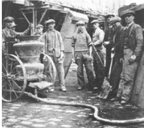
A dry-mix shotcrete (gunitite) crew in the 1920s.
