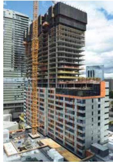
W Hotel Tower in construction.
