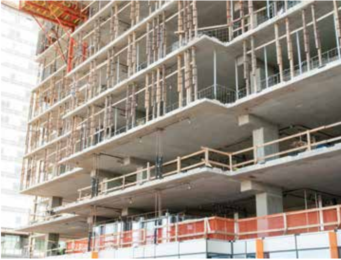
W Hotel Tower floor slabs.
