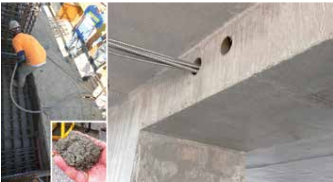
SFRC link beams.
