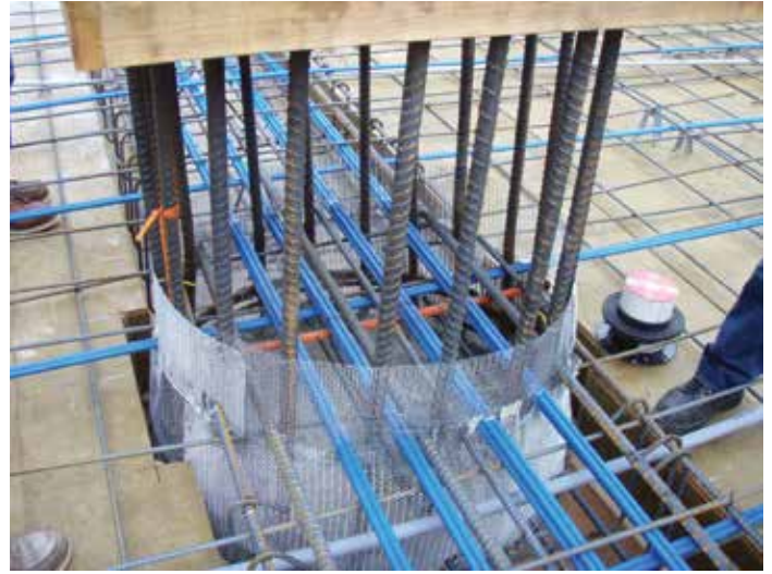
High strength column concrete placement at slab.
