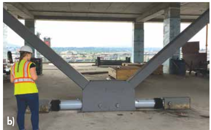
Figure 3. (a) Fluid viscous damper installation, and (b) completed braced frames with two fluid viscous dampers per V-configuration shown at floor level.
