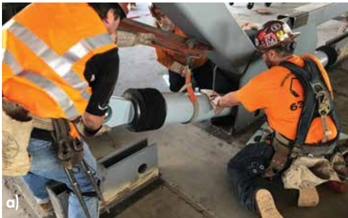
Figure 3. (a) Fluid viscous damper installation, and (b) completed braced frames with two fluid viscous dampers per V-configuration shown at floor level.
