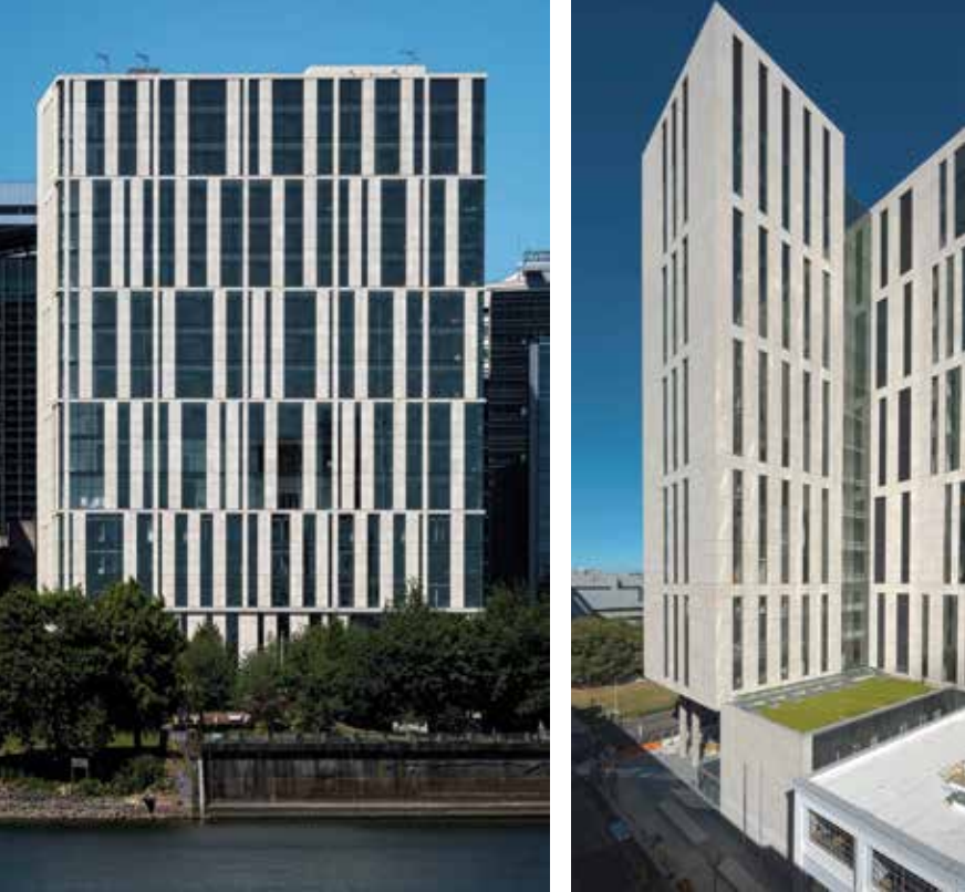
Figure 1. The completed Multnomah County Central Courthouse. Courtesy of Michael Talbot.
