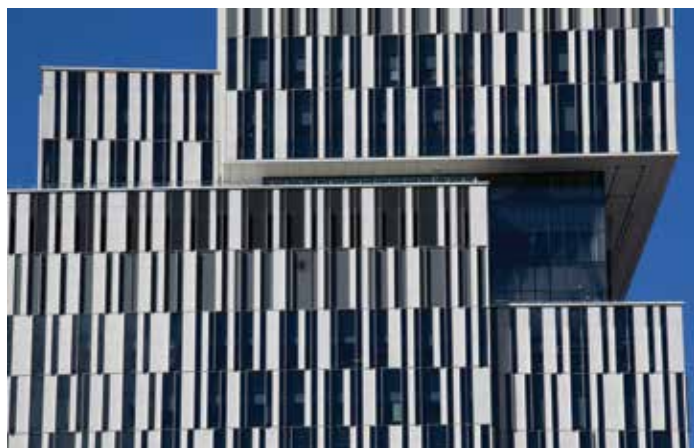
A close-up of a building setback with monorails incorporated into the soffit.
