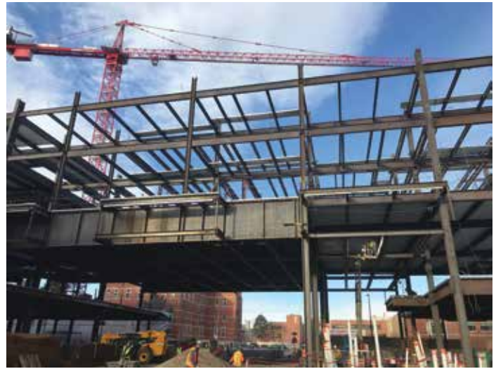
9-foot-tall plate girder spanning over Seventh Avenue.
