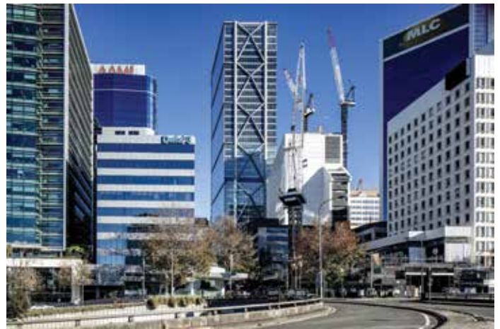
Figure 3. Eastern bracing aligned to floors at \frac{2}{3} rd point. Courtesy of Brett Boardman.
