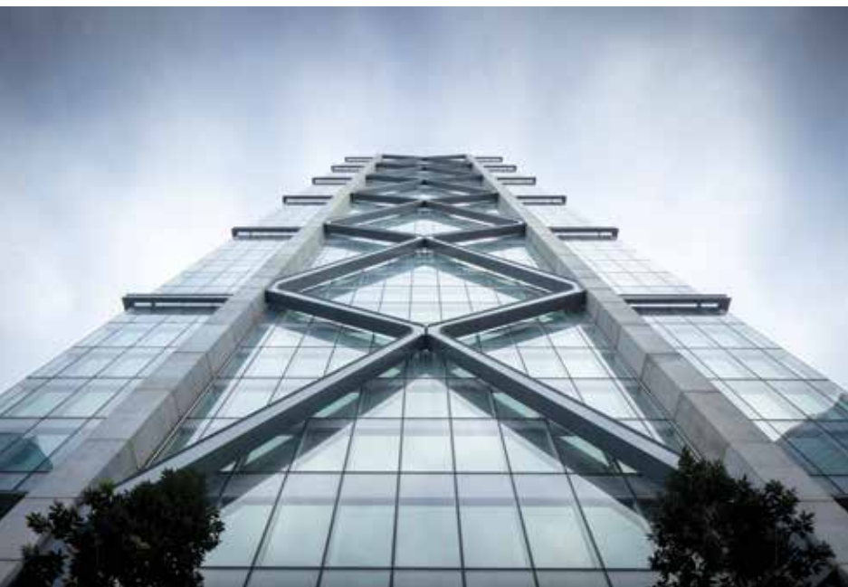
Figure 5. View of eastern mega bracing from ground level of Walker Street. Courtesy of Brett Boardman.
