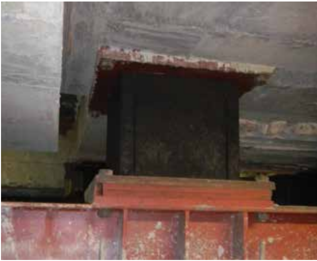
Figure 1. Seismic base isolator.
