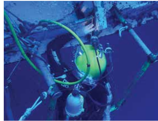
Figure 1. Welder diver performs underwater wet welding.
