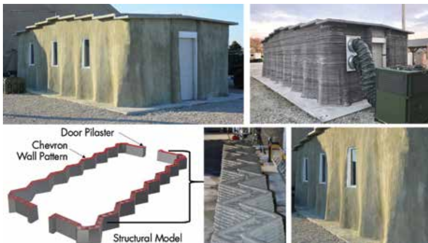
Figure 2. 3D-printed Barracks Hut. Photos courtesy of the U.S. Army Corps of Engineers. Rendering courtesy of Skidmore, Owings & Merrill.
