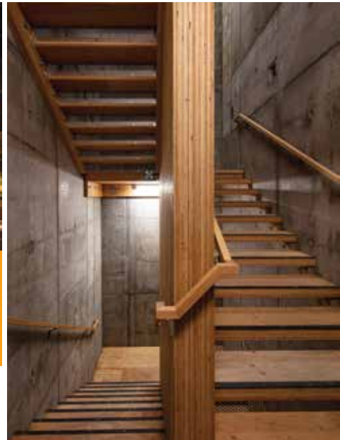
Figure 2. Stairway constructed of mass plywood.
