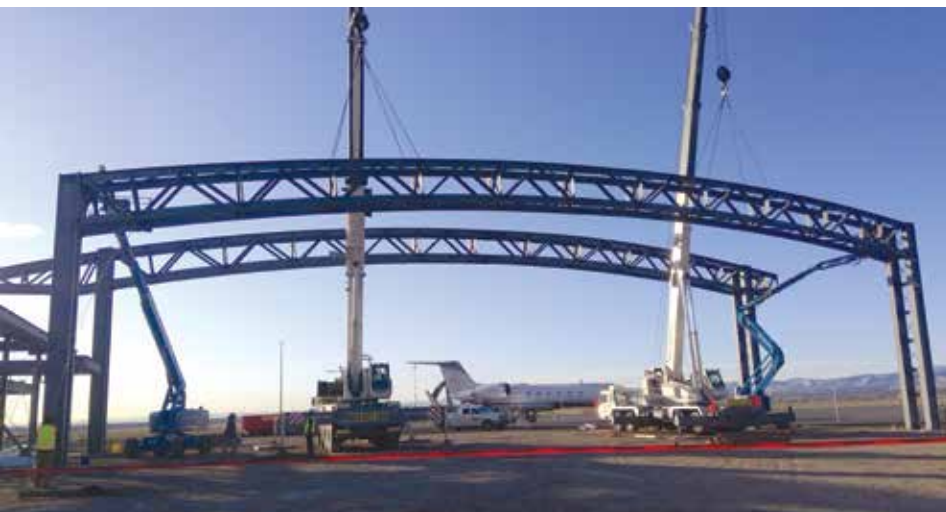
Figure 3. Two cranes were used to set the canopy trusses in place.
