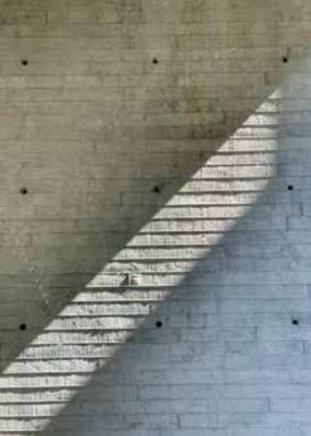
Highly textured, board-formed concrete shear walls are prominently featured throughout the completed structure.
