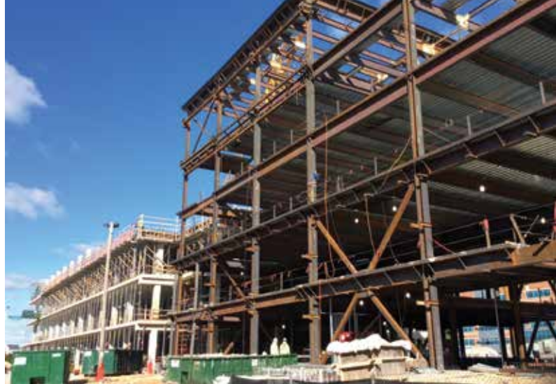
Concrete and steel are interwoven throughout Building 201 to maximize each material's structural efficiency.
