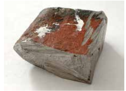
Figure 1. A sample of a wrought-iron beam flange.
