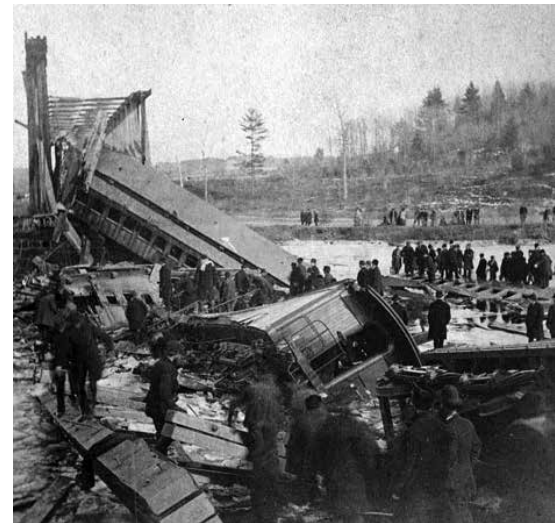
Tariffville Bridge disaster.
