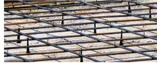
Figure 1. Slab on grade with reinforcing bars.
