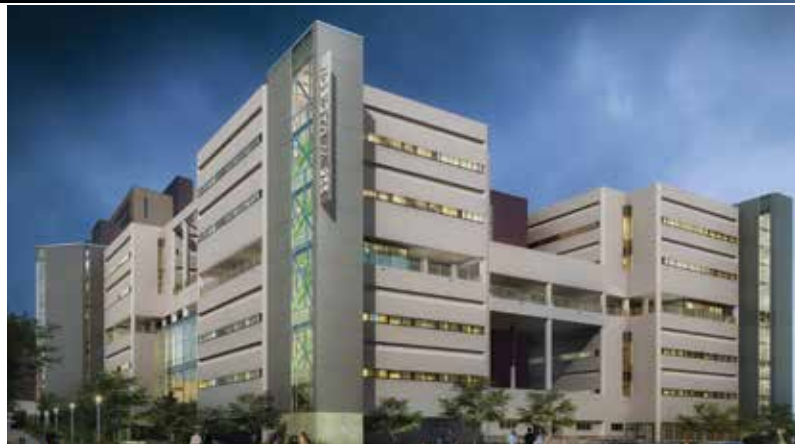
Project overview before (top left) and after (bottom) – Adaptive reuse at 225 W. Madison, formerly Madison Street Jail in Phoenix, AZ.
