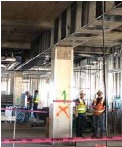
Carbon fiber polymer wrap used in shear and moment reinforcing applications.
