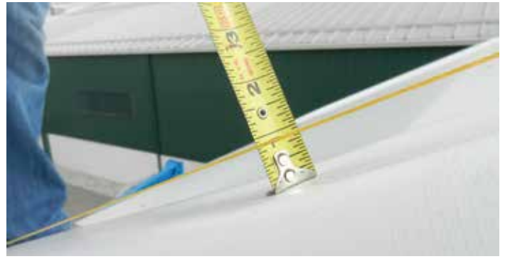
Figure 4. Steel deflection measurements collected along the length of the arch frames.
