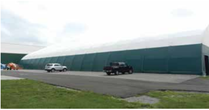
Figure 3. Overall view of the fabric shell structure.
