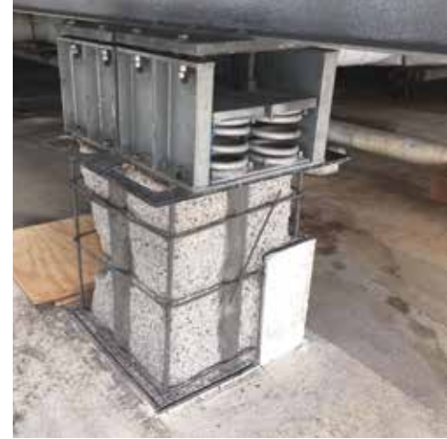
Figure 4. Repair of the concrete pedestals revealed the encased steel pipes.
