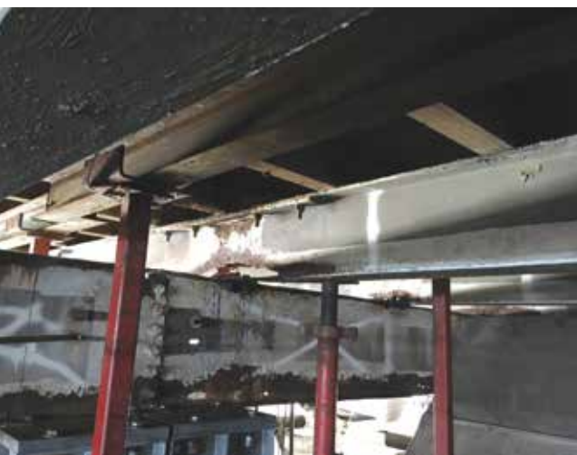
Figure 3. Post shores and horizontal shoring beam.
