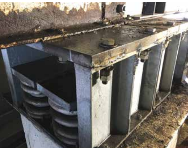
Figure 2. The base isolator bearing plate was temporarily welded.
