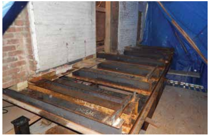
Figure 6. Needle shoring through a brick wall.
