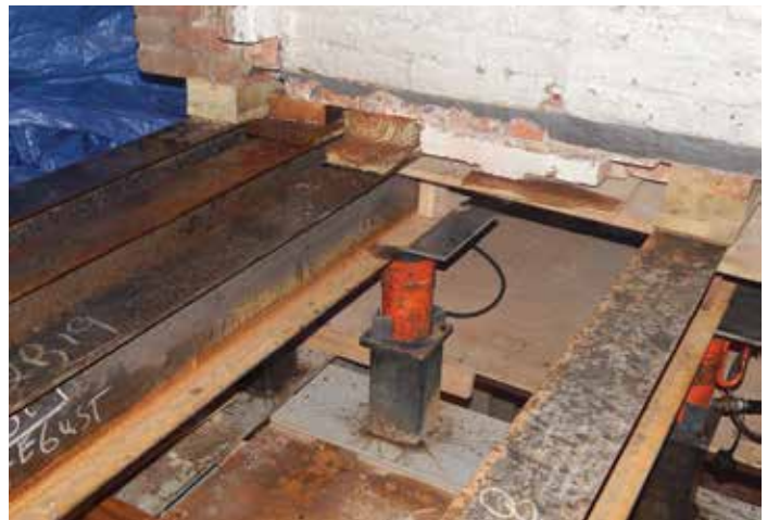
Figure 7. Needle shoring in a masonry wall with a hydraulic jack.
