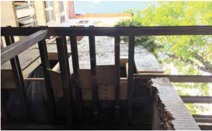
Figure 3. View looking up at a needle shoring scenario.
