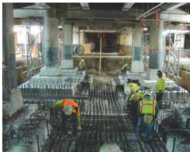
Figure 4. Crews install foundation reinforcement at the bottom of the new mat foundation. Notice “wedding-cake” style original concrete foundations at varying elevations.
