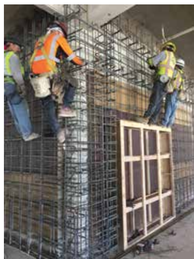
Figure 3. Reinforcement installation at new shear wall core. Note doweling to the existing corner column and force-transfer bolts into the existing girder at the top of the wall.
