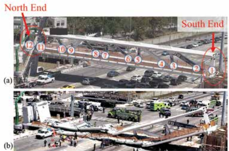
Figure 1. Main span of the bridge: a) before collapse; b) after collapse. Courtesy of NTSB.
