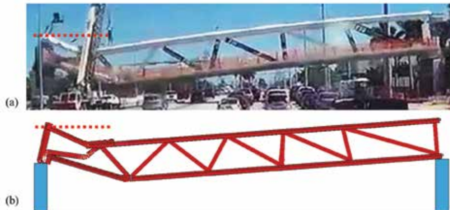
Figure 5. Failure mode of the bridge from a) accident video frame, courtesy of Instagram/@o2webdev; and b) computer simulation.
