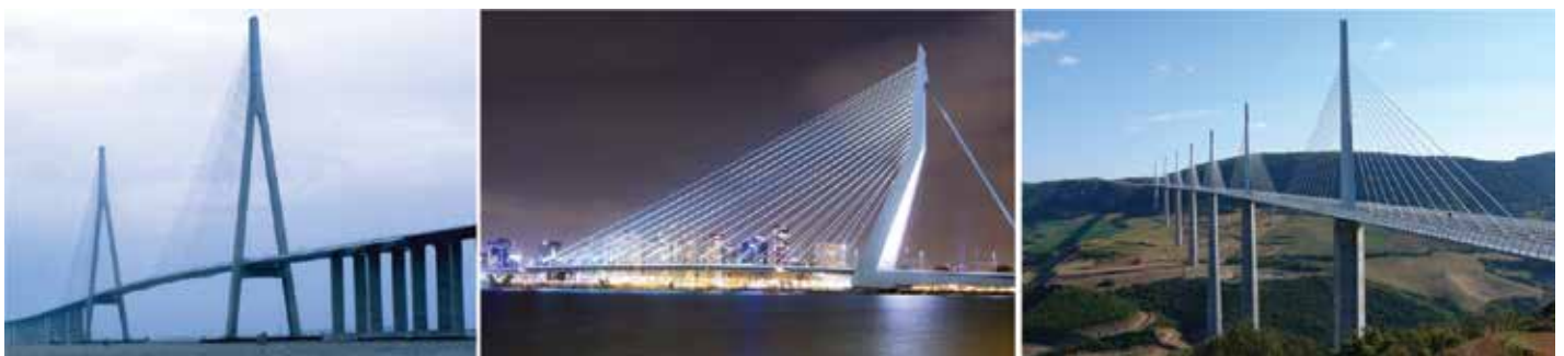
Figure 2. Span options: main with two sides spans, asymmetric and multi-span.
